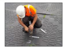
Please be sure not to over tighten bolts, as this can cause cross-threading and damage to the connectors.
